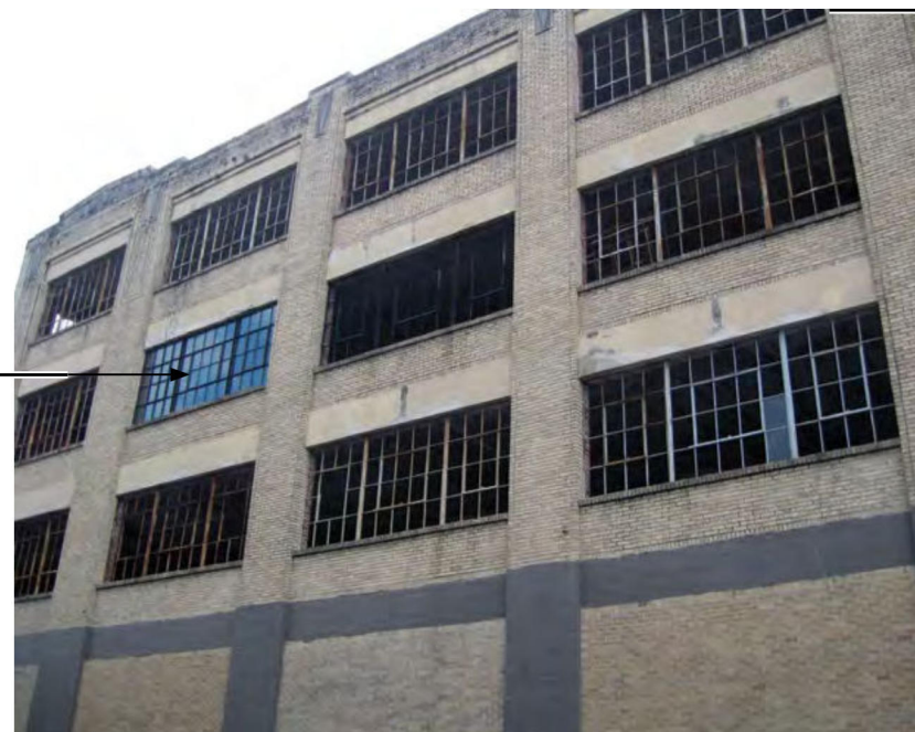
[19] Installing a mockup of a proposed replacement window can be helpful to evaluate how well the new windows will match the historic windows that are missing or too deteriorated to repair.
