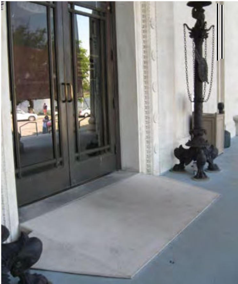
[26] A temporary ramp-unobtrusive and easily removed-facilitates access to the entrance of this museum and does not affect its historic character.
